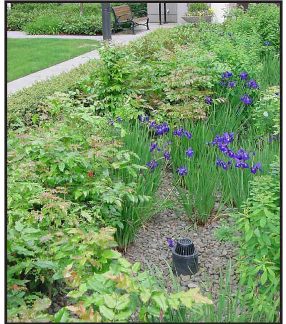
Figure 6.2 Infiltration Basin. Source: David Dods
