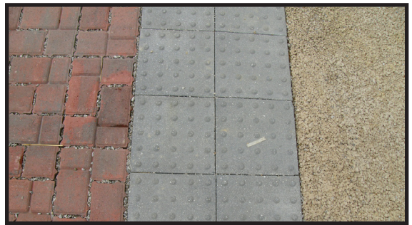
Figure 6.27 Pervious pavement types. Source: Williams Creek Consulting.
