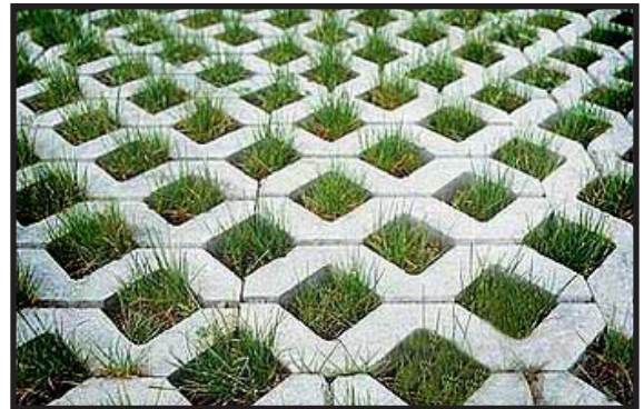
Figure 6.24 Turf pavers. Source: Williams Creek Consulting.
