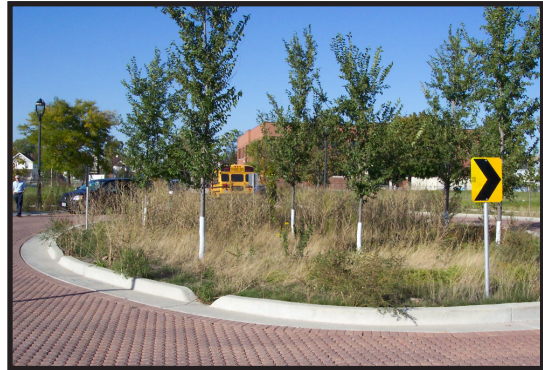
Figure 2.13 Rain garden in roundabout designed to capture/ infiltrate stormwater, Milwaukee, WI. Source: Bob Newport, EPA Region 5
