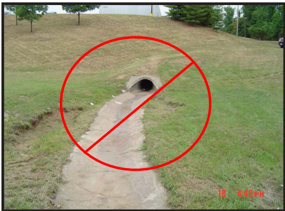
Figure 6.55 Detention basin with concrete conveyance channel. Source: Metropolitan St. Louis Sewer District
