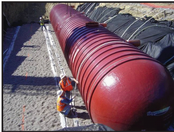
Installation of the water harvesting cisterns.
