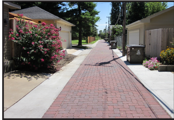
Figure 1.9 Pervious alley in St. Louis City. Source: Metropolitan St. Louis Sewer District
