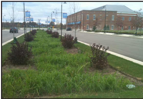
Figure 6.32 Bioretention - Delaware Health Village, Delaware, OH. Source: Williams Creek Consulting
