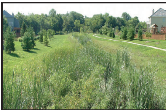
Figure 5.5 Wetland Swale. Source: Olsson Associates
