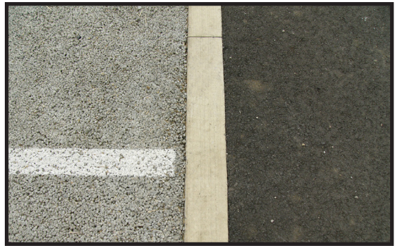
Figure 6.26 Pervious concrete and asphalt. Source: Williams Creek Consulting.
