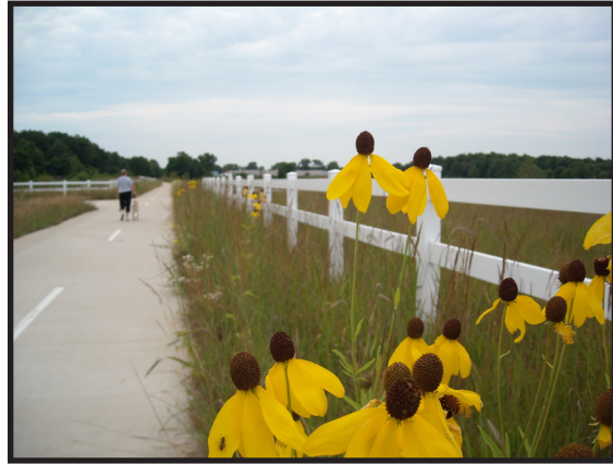
Earl Road flood control facility. Photo Source: Williams Creek Consulting.
