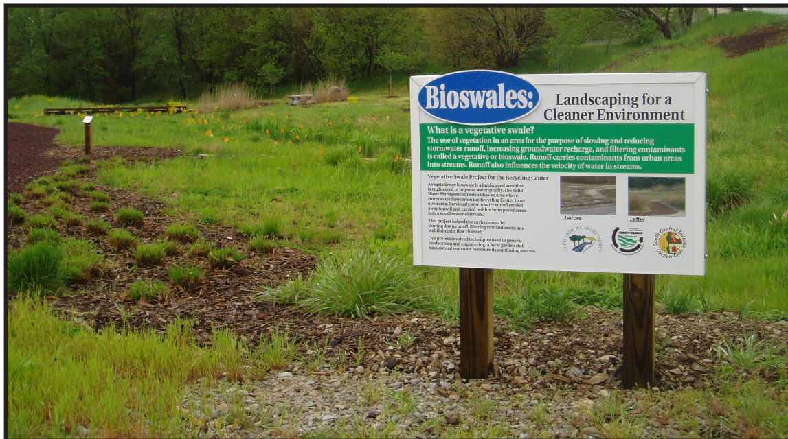
Figure 6.41 Bioswale - Clifty Creek, Ind. Source: Williams Creek Consulting.
