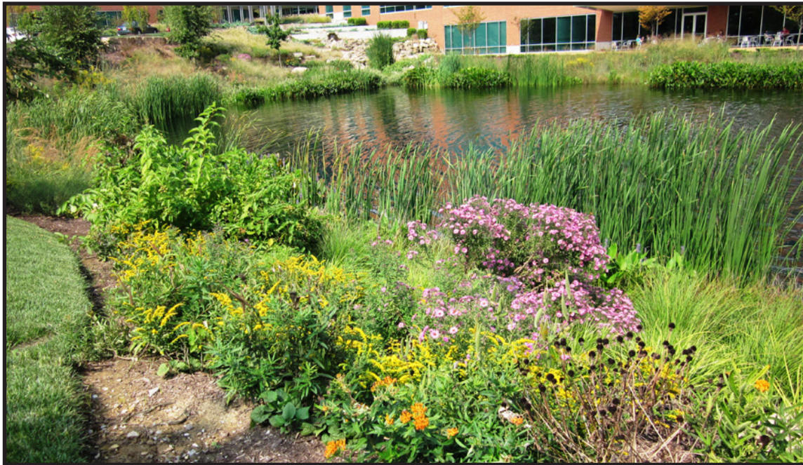
Figure 6.1 Extended Wet Detention, Express Scripts Campus, Berely, MO. Source: Metropolitan St. Louis Sewer District.
