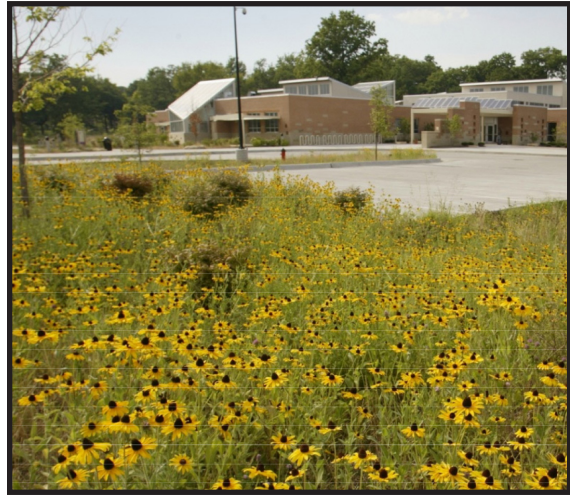
Figure 1.11 Native parking lot bioswale. Anita B. Gorman Conservation Discovery Center - Kansas City, Missouri. Source: Copyright © Missouri Conservation Commission. All rights reserved - used with permission.
