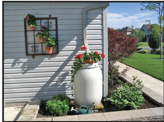
Figure 2.14: Residential rain barrel. Source: ABCs of BMPs
