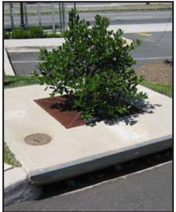
Figure 6.31 Tree vault, Arlington, VA. Source: www.arlingtonva.us/departments/EnvironmentalServices
