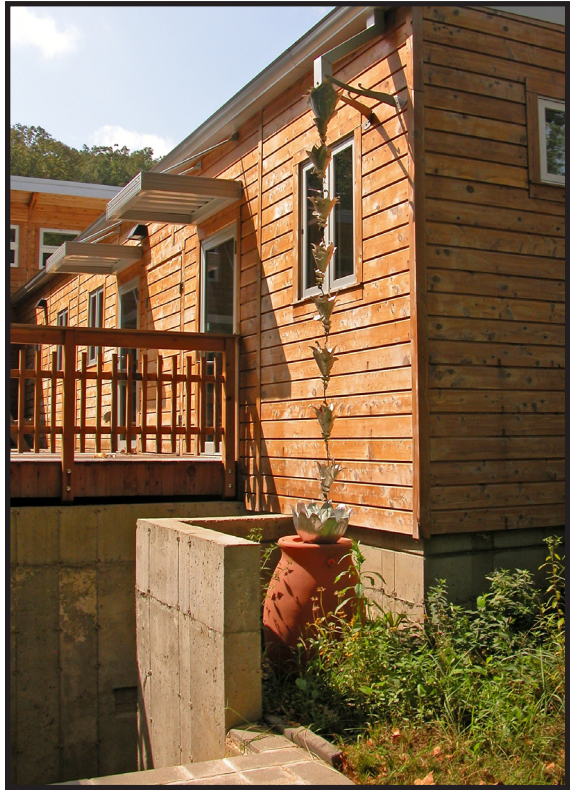
Figure 6.11 Tyson Learning Center, Washington University, Eureka, MO. Source: Williams Creek Consulting
