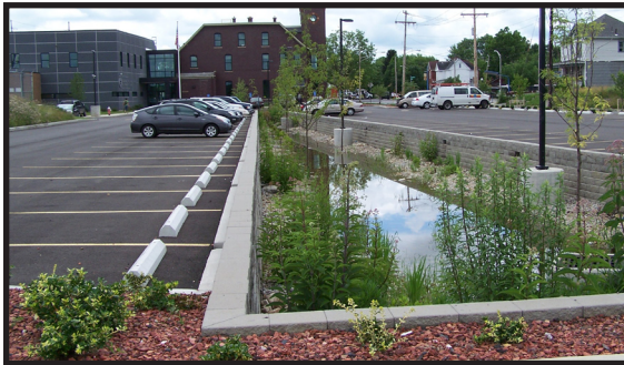
Figure 6.33 Bioretention System - medical facility in Ohio. Source: Williams Creek Consulting
