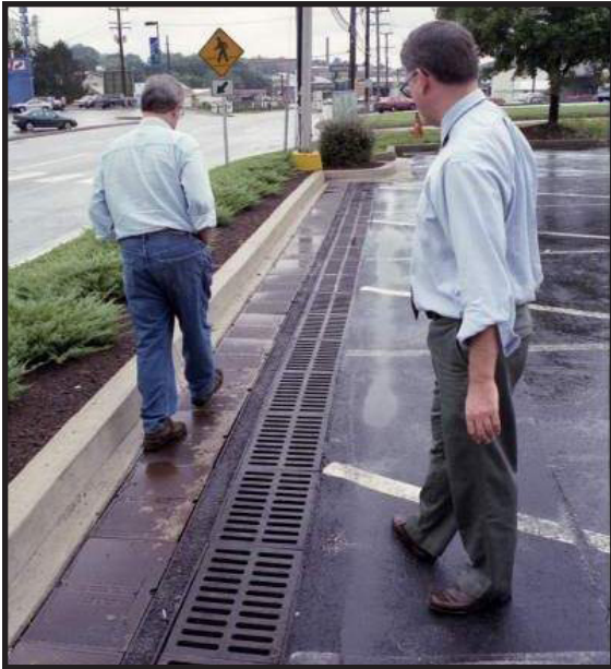
Figure 2.7 Perimeter sand filter. Source: Center for Watershed Protection
