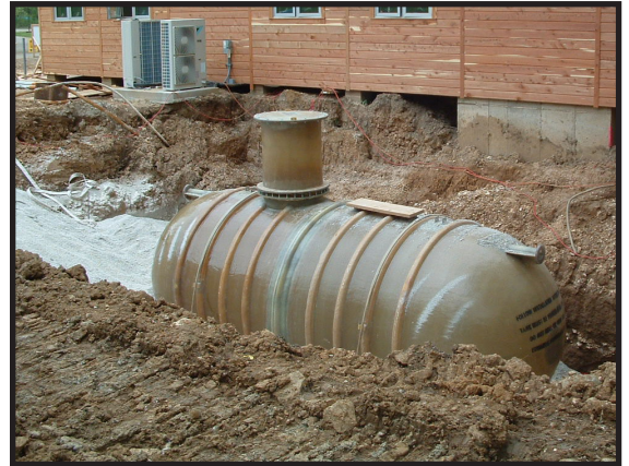
Figure 6.13 Tyson Learning Center, Washington University, Eureka, MO. Source: Williams Creek Consulting
