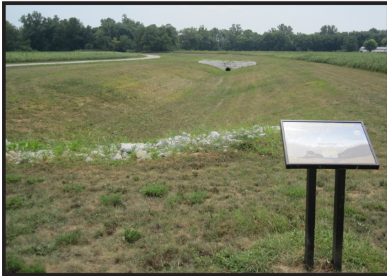
Figure 6.60 Dry Detention- Shelbyville, IN. Source: William Creek Consulting.
