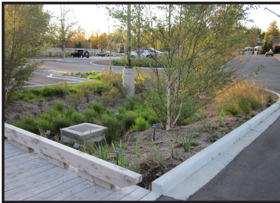
Parking lot with rain garden and overflow, plus permeable pavement and curb cutouts above. Source: Metropolitan St. Louis Sewer District
