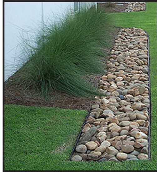
Figure 6.18 Infiltration Trench - Bellingham, WA. Source: Williams Creek Consulting.
