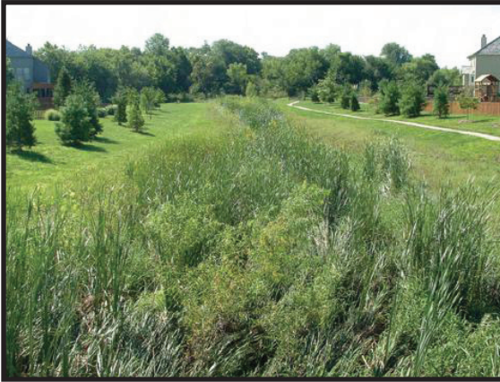
Wetland Swale. Source: Olsson Associates
