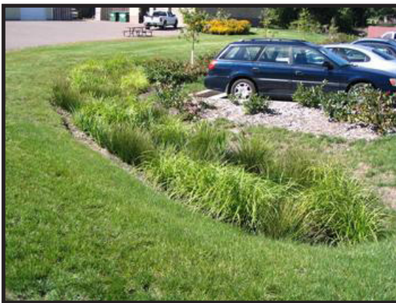
Figure 2.19 Vegetated Swale - MN. Source: Ramsey-Washington Watershed District - BMP Descriptions
